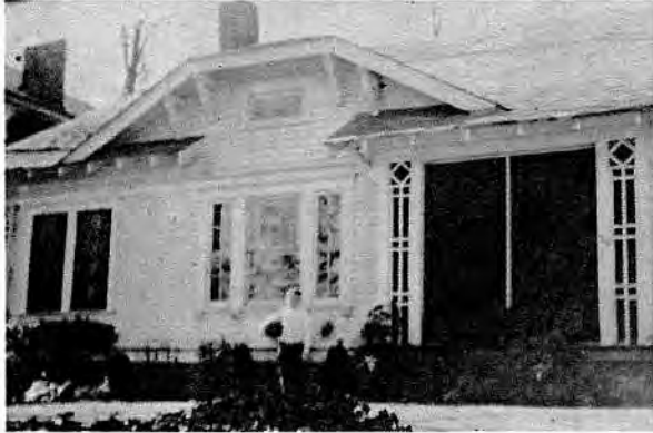
This photo, provided by Wilburn's niece, shows one of her houses. It was among many demolished to build Decatur's Carl G. Renfroe Middle School in the early 1970s.
